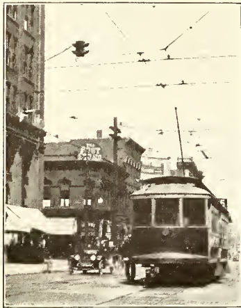
HEAT CONTROL SIGNAL INSTALLED IN HEART OF DENVER
